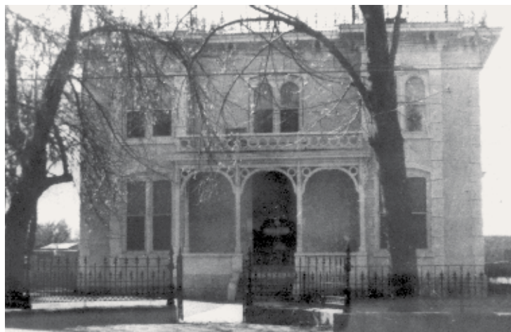
The Staab House, after the fire
